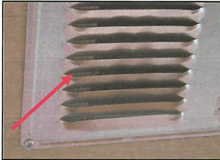
Figure 10. The 1/8" screening can be seen where it contrasts with the wood on the left side of the vent.
